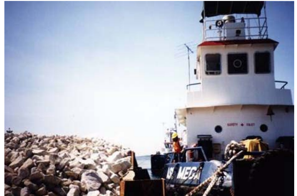
Transport of rocks for pipeline system
